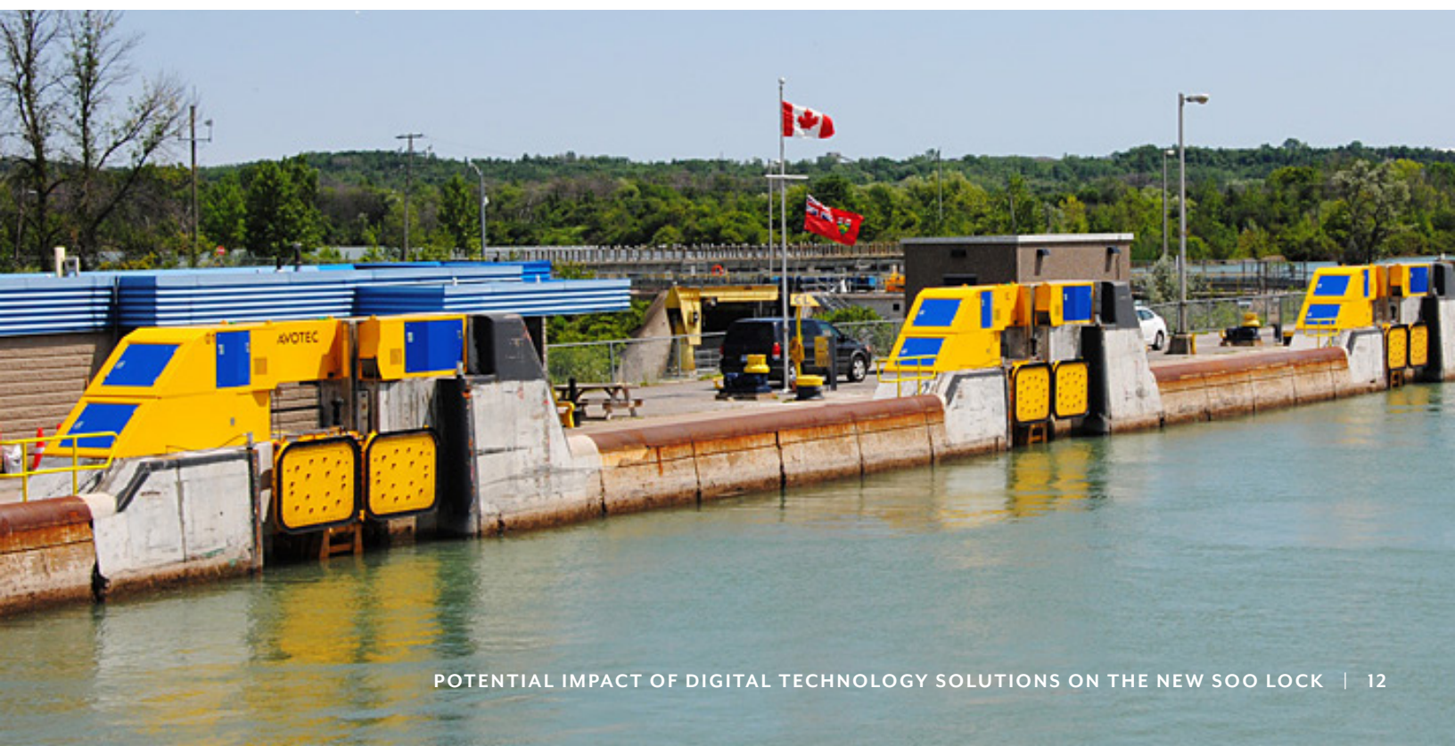
Figure 3. Illustration of Hands-free Mooring from the St. Lawrence Seaway (Image courtesy of the GLS)
